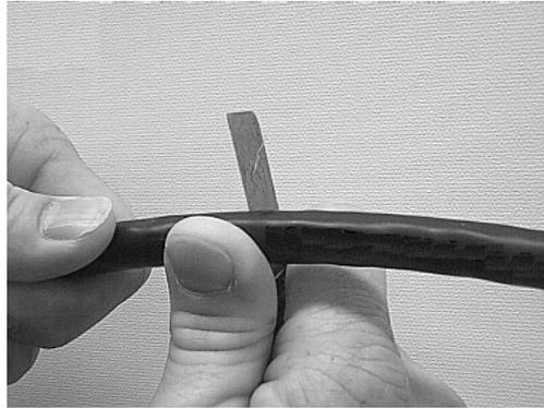
**Figure 21 – Ring cut the cable jacket.**
