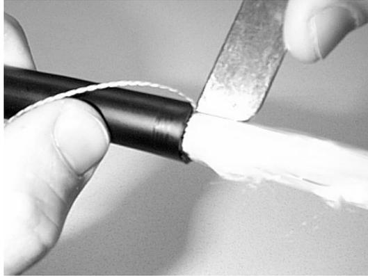
**Figure 6 – Cut a starting slit adjacent to the rip cord.**
