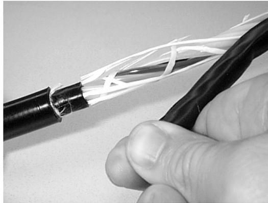
**Figure 15 - Remove the inner cable jacket.**
