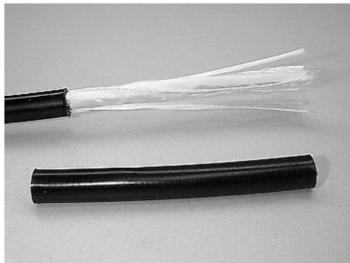
**Figure 13 - Remove the 5-inch section of inner jacket.**
