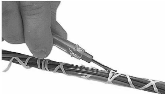
**Figure 16 - Remove the binder threads and water blocking tape.**
